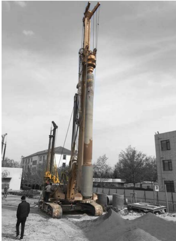
Piling for hole drilling diameter 1m, depth 30m with 3xLUY390x30
